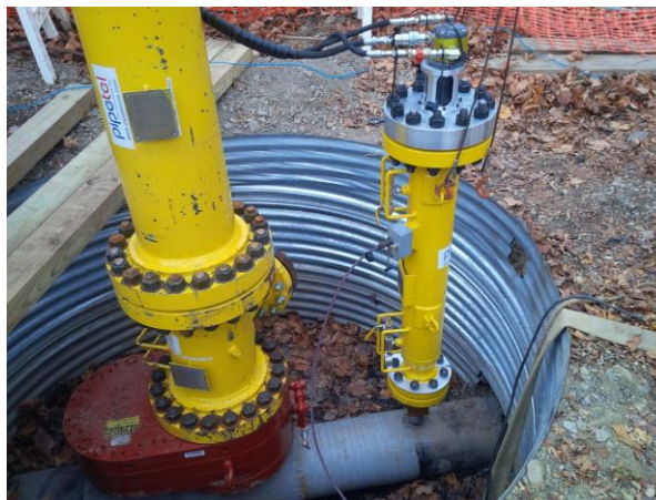
Figure 4: In-line Charging Tool in Live Setup
